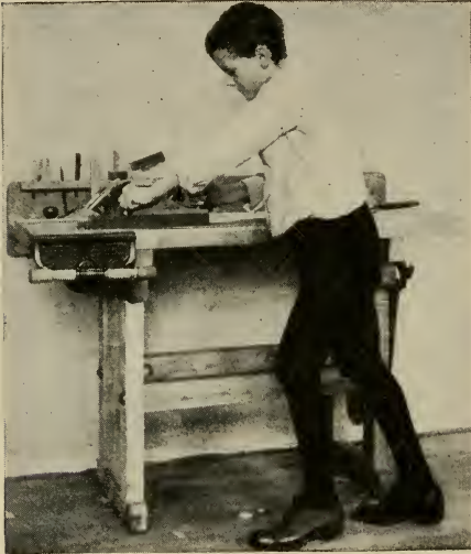
Fig. 9—Position for Planing
